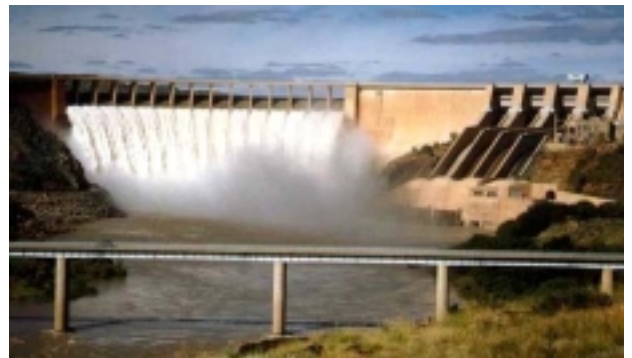
Kloop Dam: part of the infrastructure handed over to the ANC.
