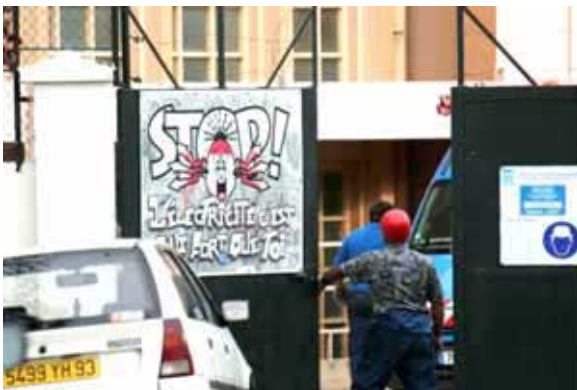
The gate to the sub-station where the boys were electrocuted. The sign says "Stop! Electricity is stronger than you are."
