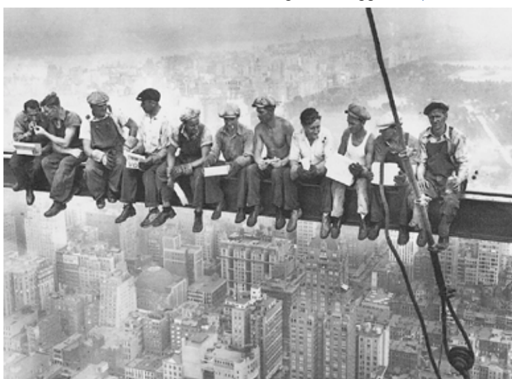
Lunchtime for the ironworkers on the Empire State Building.
