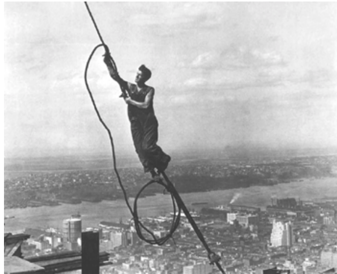
Working on the Empire State Building.
